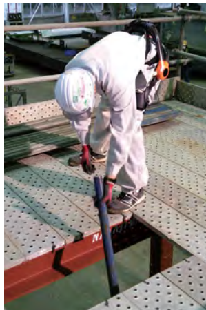
Assembling temporary scaffolding
