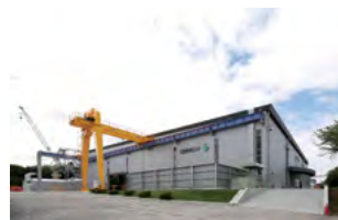
Exterior of the Osaka Machinery Plant maintenance building
