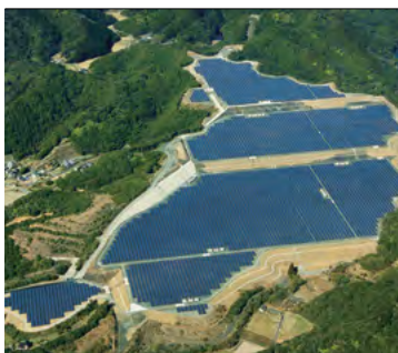
Hyugahichiya Solar Power Station
