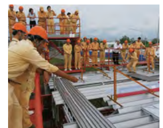
Trainees learning how to install a roof
