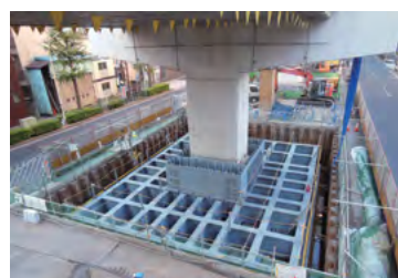
Hybrid structural footing framework
