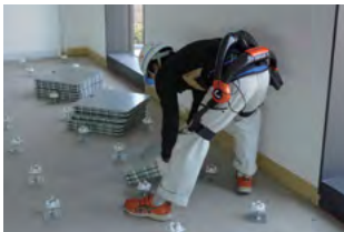
Installing a raised floor
