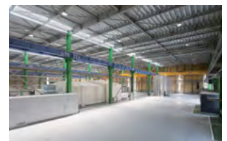
Expanded BCP functions include emergency power generators, an emergency supply warehouse, etc.
