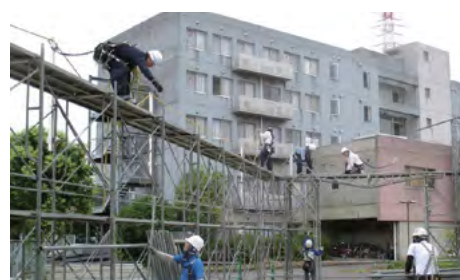
Learning to assemble scaffolding by doing the actual work
