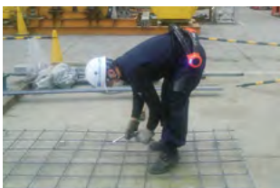
Tying down floor rebar
