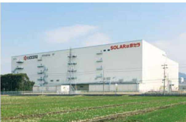
Kyocera Shiga-Yasu Factory Building No. 28 ('10) Location: Yasu, Shiga
