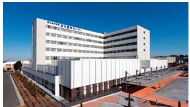
National Hospital Organisation Yokohama Medical Center ('10)
