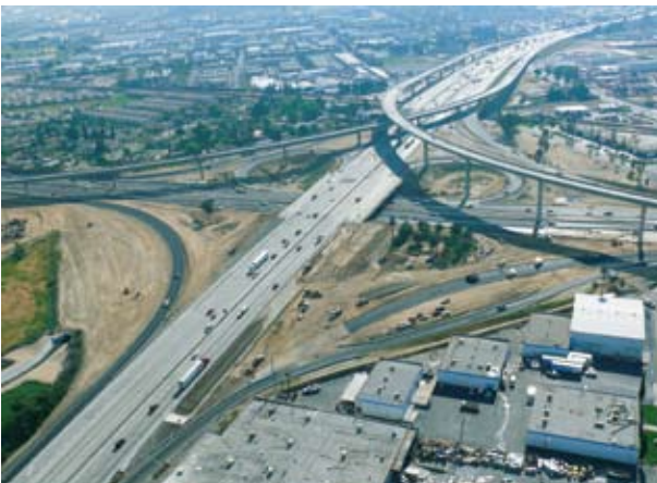
60/91/215 Corridor Improvement Project ('08) Location: Riverside, California, U.S.A.
