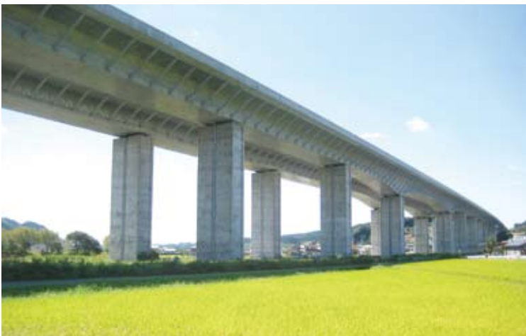
New Tomei Expressway Miyagashima Viaduct ('10)
