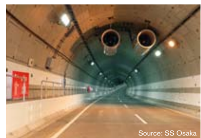
Hanshin Expressway Inariyama tunnel ('09) Location: Kyoto
