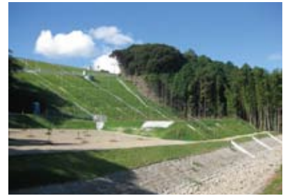
Restoration of Tomei Expressway in Makinohara ('10) Location: Shimada and Makinohara, Shizuoka
