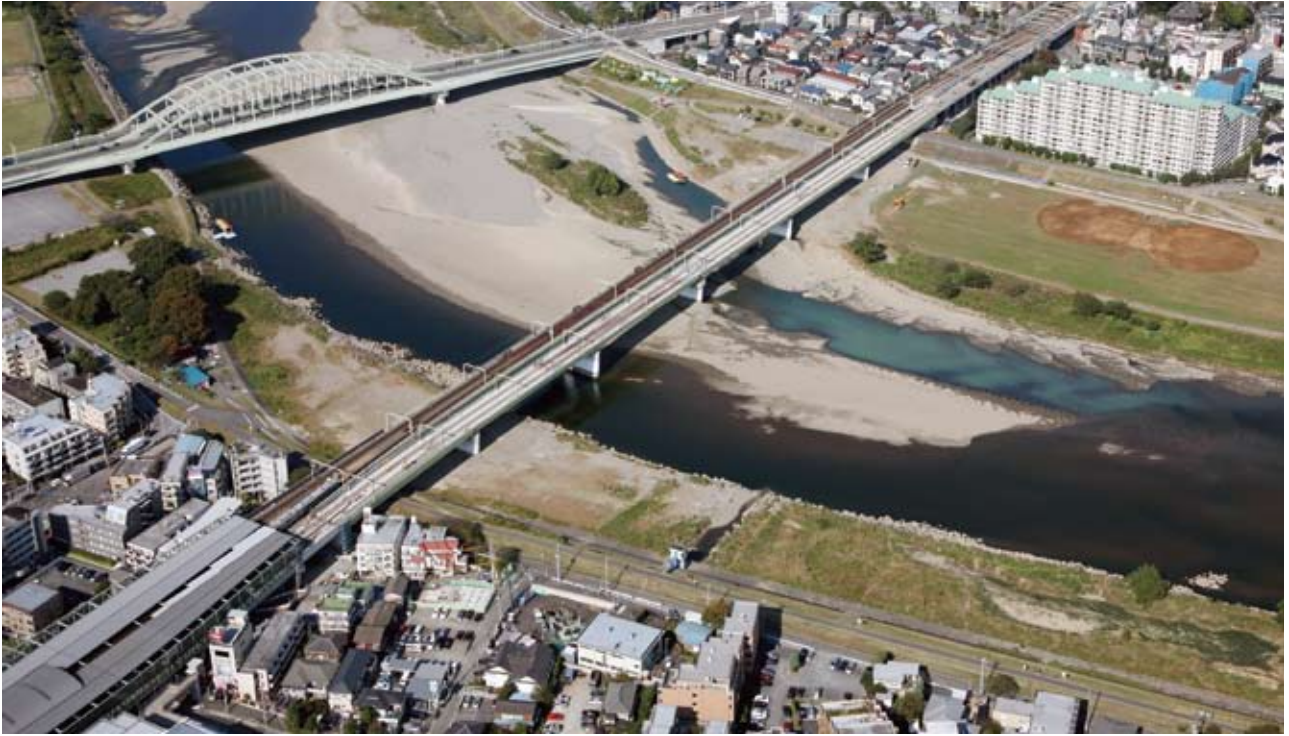
Odakyu Electric Railway Tamagawa Bridge ('10)
