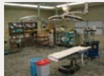
Operating room (before renovation)
