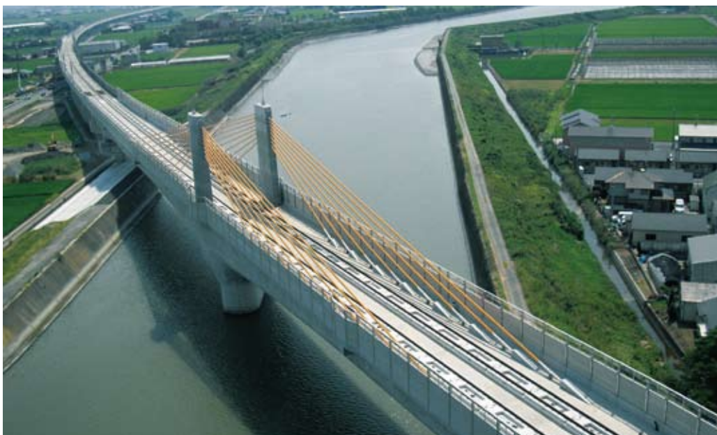
Kyushu Shinkansen Onogawa Bridge ('09) Location: Uki, Kumamoto
