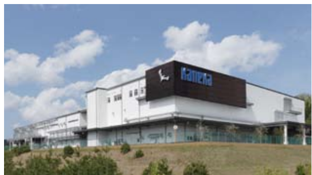
Kaneka Solartech Factory No. 2 ('09) Location: Toyooka, Hyogo
