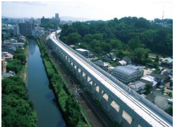
Kyushu Shinkansen Kitaoka Viaduct ('09) Location: Kumamoto, Kumamoto
