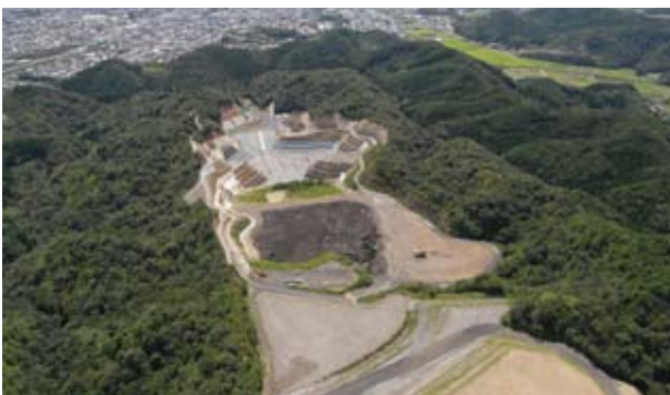
Processing Plant of Secondary Slag in Tsurunouchi ('10)
