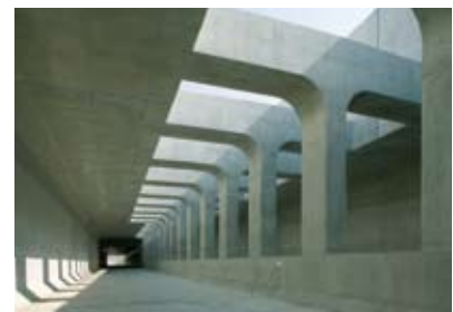
Higashi Meihan Expressway Hirabari Excavation Tunnel ('09) Location: Tempaku-ku, Nagoya
