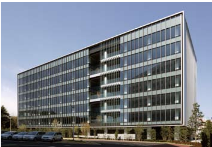
Heiwajima Tosei Building ('10)
