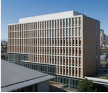
Taisho University Building No. 7 ('10) Location: Toshima-ku, Tokyo
