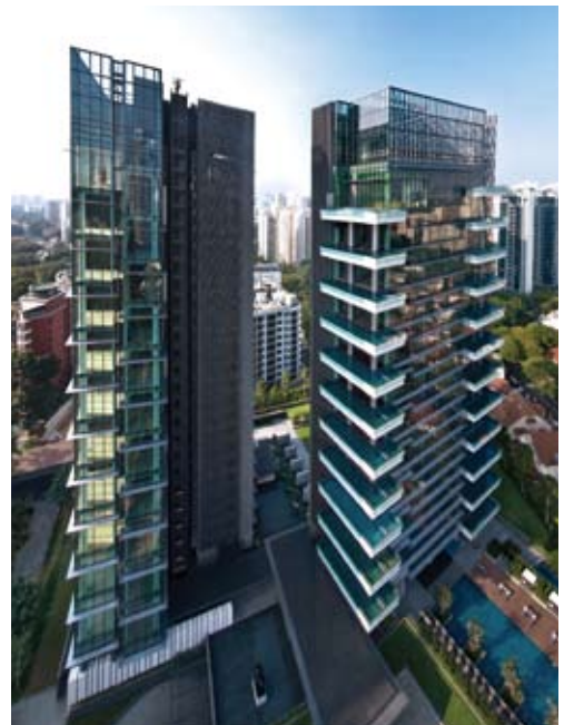
Paterson Hill Condominium ('10) Location: Singapore
