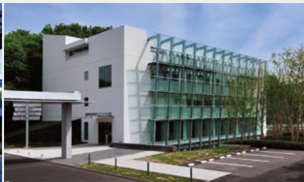
Materials and chemical engineering laboratory
