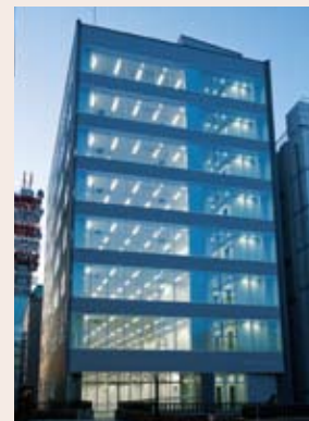
Mito North Front Building (Mito, Ibaraki)
