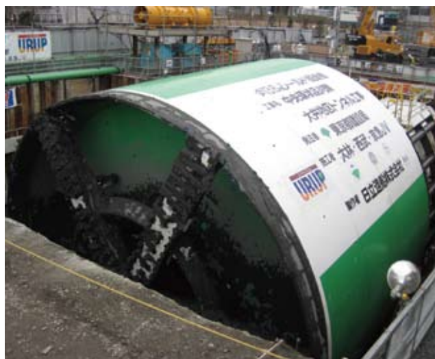
The shield machine being launched at ground level
