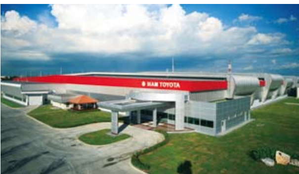
Siam Toyota Manufacturing Engine Plant No. 2 ('09)* Location: Chonburi, Thailand
