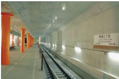
Tokyo Metro Fukutoshin Line Shinjuku 3-chome Station ('09) Location: Shinjuku-ku, Tokyo
