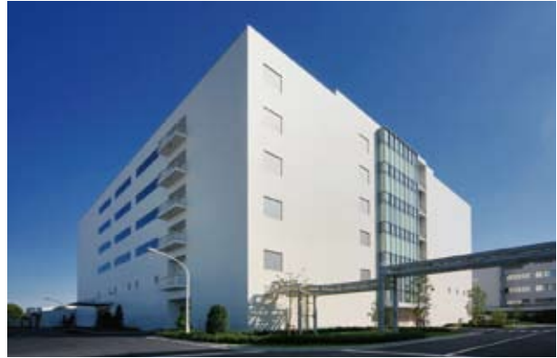
NEC Fuchu Factory ('09) Location: Fuchu, Tokyo
