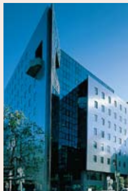
Oak Ikebukuro Building (Toshima-ku, Tokyo)
