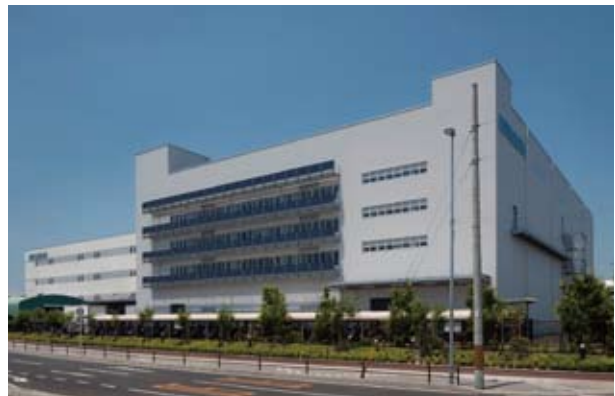
Mitsubishi Electric Corporation Air Conditioning and Refrigeration System Factory No. 7 ('10) Location: Wakayama, Wakayama
