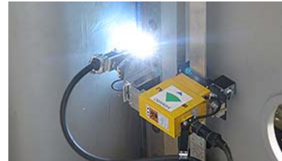
[Site Robot Welding Method]
