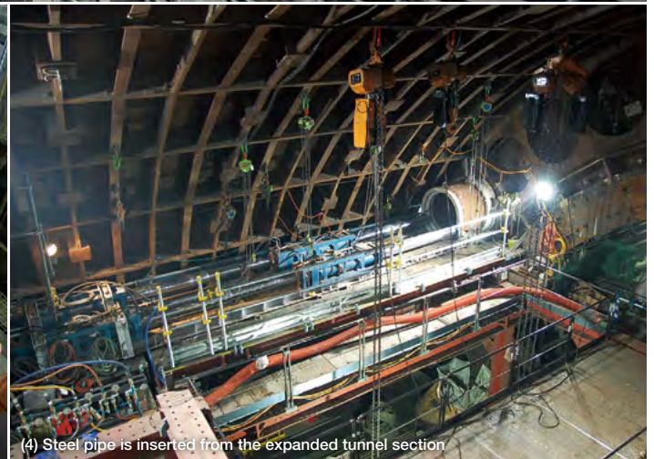
(3) Tunnel expansion shield machine is installed in a launching pit below the main tunnel
