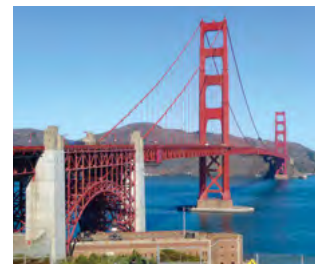
Golden Gate Bridge Seismic Retrofit (U.S.)
