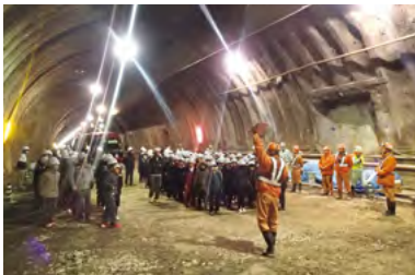
Obayashi engineers teach children how tunnels are built while walking along the site
