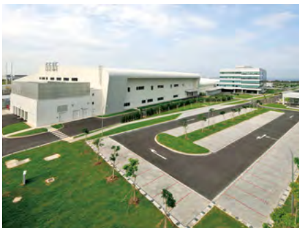
Halliburton Completion Technology and Manufacturing Center (Singapore)
