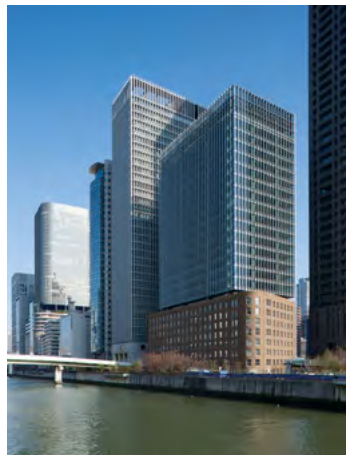
Daibiru Honkan Building
