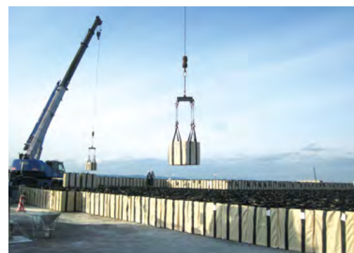
Upcycle Blocks stockpiled for use in earthquake reconstruction projects
