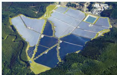
Ashikita Solar Power Station (Ashikita District, Kumamoto Prefecture)
