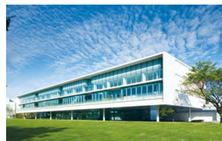
Obayashi Technical Research Institute Main Building
