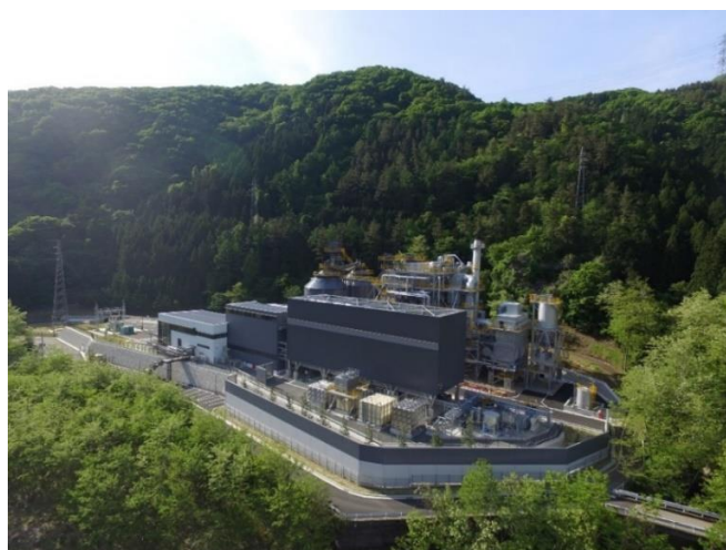
[Project 03-2 Otsuki Biomass Power Plant]
