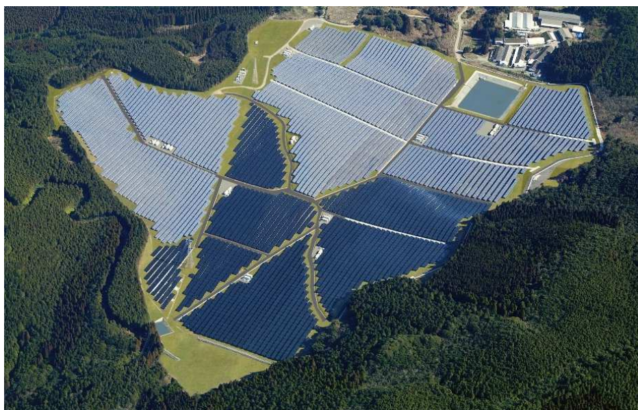
Project 01 Ashikita Solar Power Station, Solar PV
