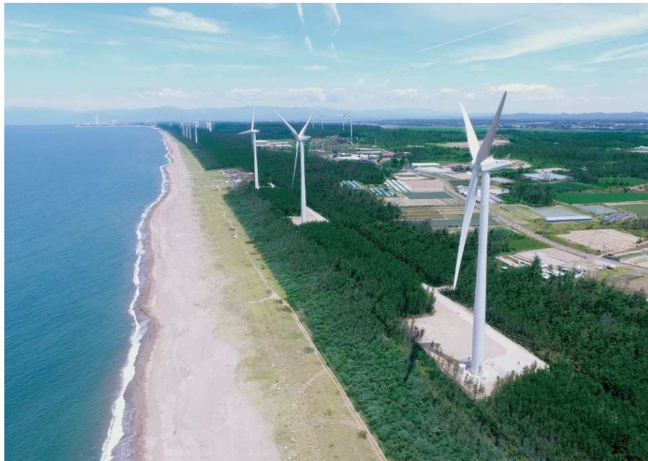
Project 04 Mitanehamada Wind Power Station
