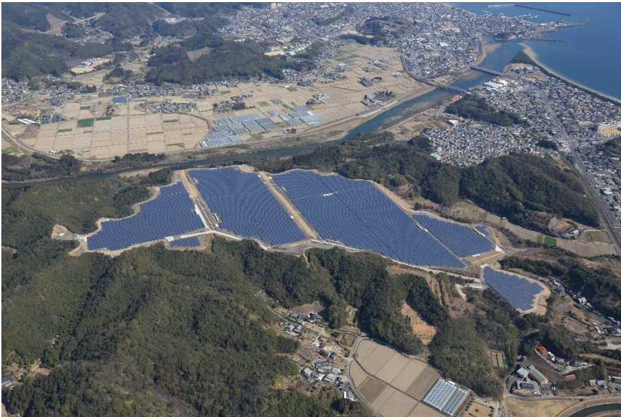
Project 03 Hyugahichiya Solar Power Station, Solar PV
