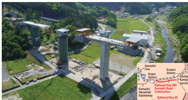
National Highway 45 Yoshihama-Kamaishi Road Construction (Toni Viaduct Bridge No. 2, Arakawa Tunnel)
