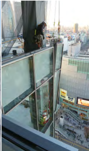
Attaching the curtain wall using the outer wall lifting system
