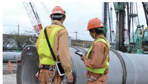
Recording inspection result data on a tablet
