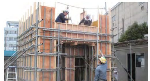
Participants practicing assembling formwork
