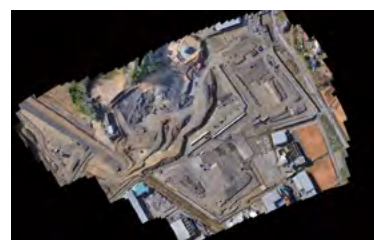
Multiple photos are used to create an image of the entire construction area
