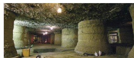
Existing underground piles supporting the METI building
