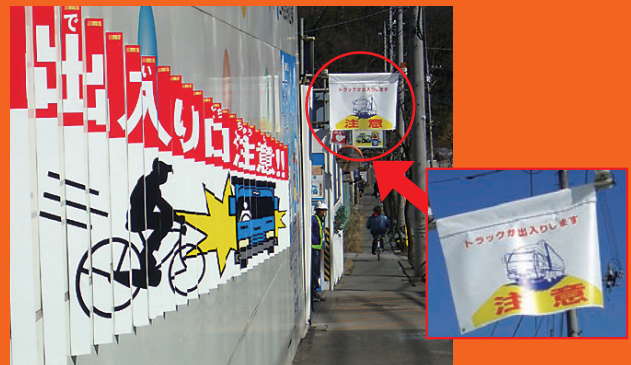
To prevent construction vehicle accidents involving pedestrians, we erect signs with lights, sounds and crossing bars to attract people's attention
