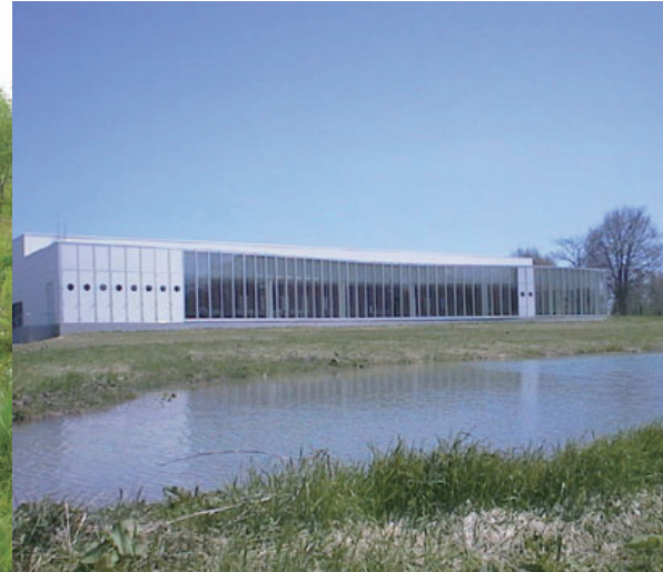
The north side view of the Nakatsunai Plant The pond utilizes spring water
