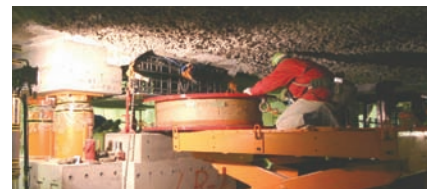
Replacing with new seismic isolators
