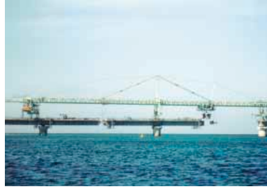
A long bridge being built with a balanced cantilever system.
