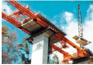
A medium-sized bridge takes shape span by span.
