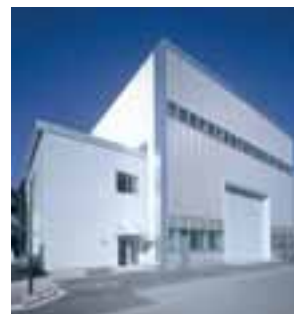
Fire Protection Engineering Laboratory
