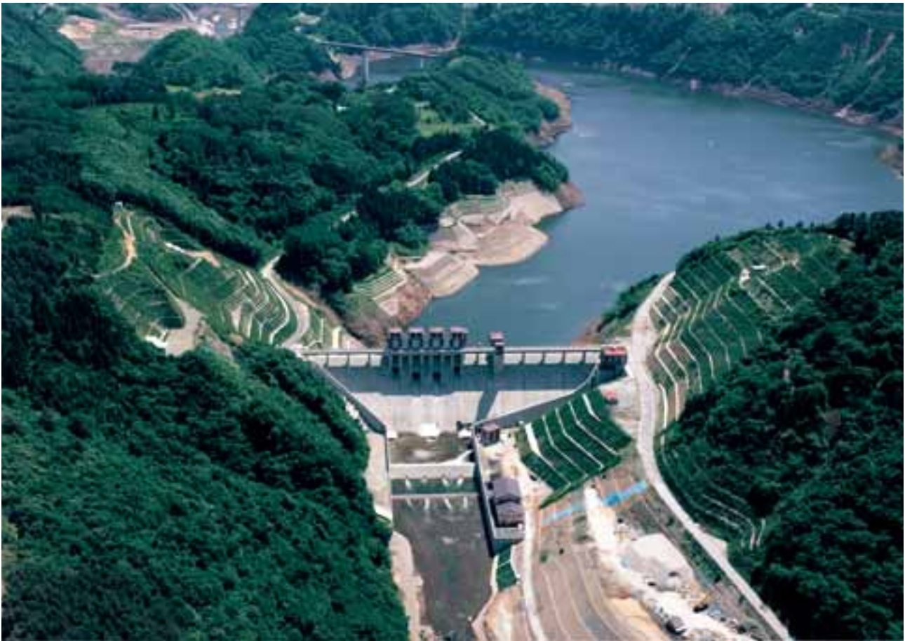
Yomasari Dam Location: Aomori
