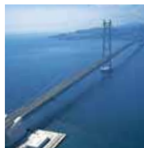
Akashi Kaikyo Bridge (Kobe Side Anchorage)
