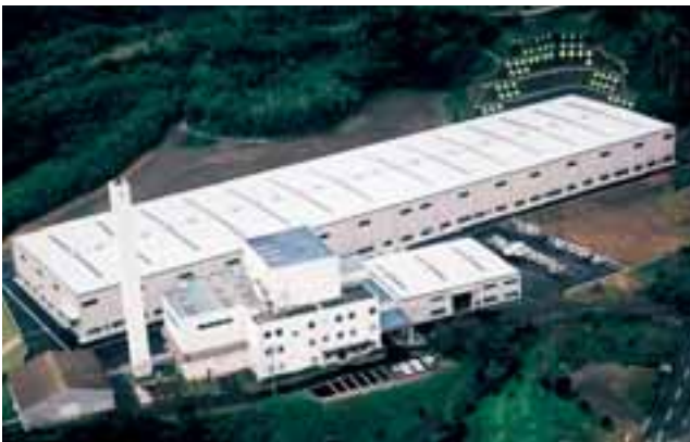
Usuki City Disposal Factory Location: Oita
