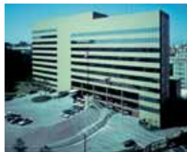
U.S. Embassy Office Building
