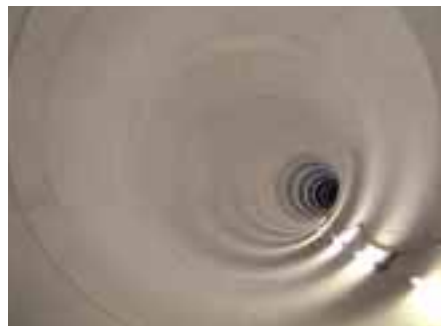
Otai Reservoir Tunnel Location: Aichi
