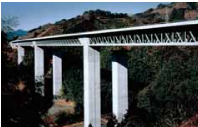
The Second Tomei Expressway Sarutagawa-bridge and Tomoegawa-bridge Location: Shizuoka
