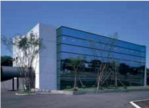
The Main Building (The Super Energy-Conservation Building)
