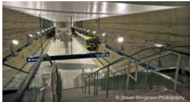
MSP LRT Tunnel and Station Location: Minnesota, USA
