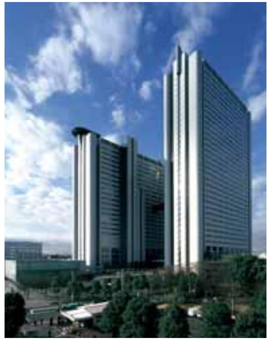
Hall (front, far left), North Tower (right) NEC Corporation Tamagawa Renaissance City North Tower / Hall Location: Kanagawa
