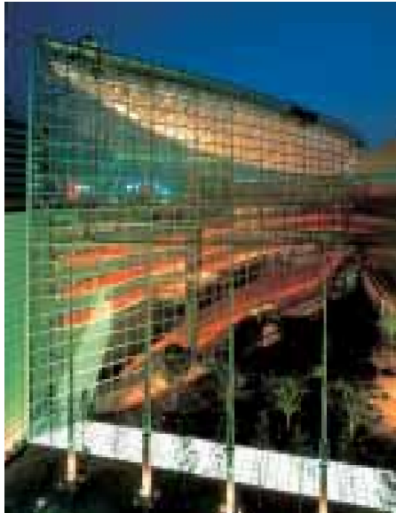
Tokyo International Forum Glass Hall Completed in 1996
