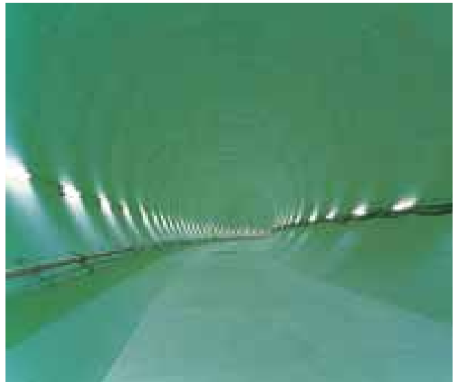
The Metropolitan Area Outer Discharge Channel-Tunnel Contract No.1
