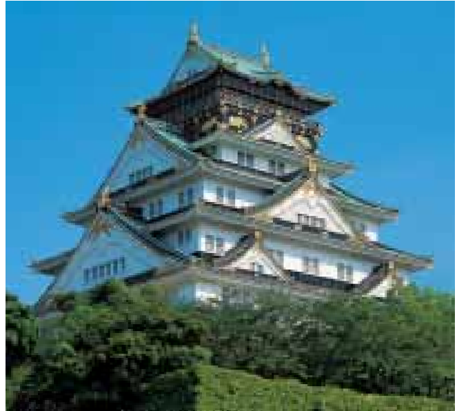
Osaka-jo Castle "The retrofit work of Heisei"
