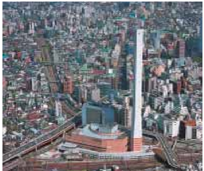
Toshima Incineration Plant
