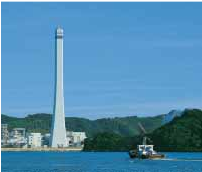
Shikoku Electric Power Co., Inc. Tachibana-wan Thermal Power Station, Chimney
