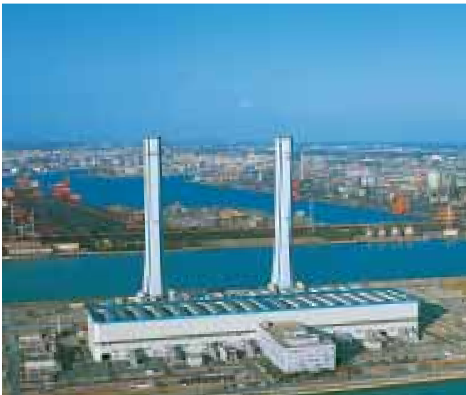
Tokyo Electric Power Co., Inc. Chiba Thermal Power Station
