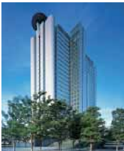
NEC Tamagawa Renaissance City (I)
