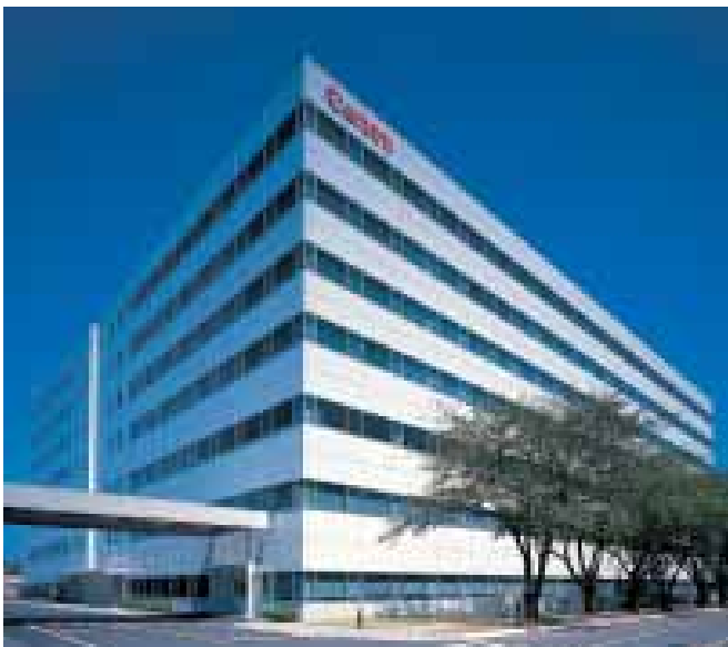
Canon Inc. Toride Plant 98A-B-1 Building
