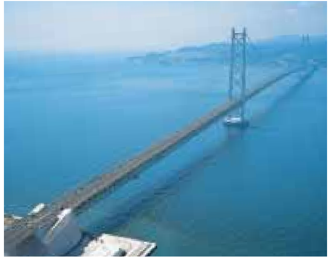
Akashi Kaikyo Bridge (Kobe Side Anchorage)
