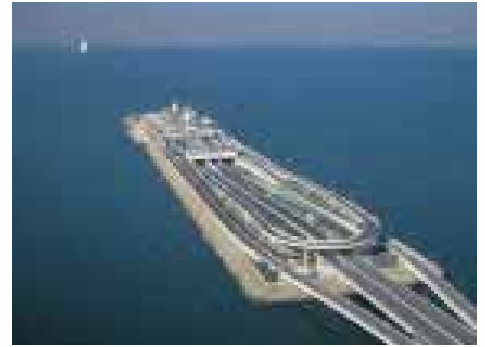
Tokyo Wan Aqua-Line Completed in 1997
