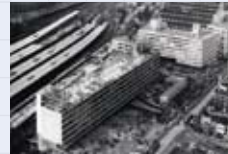
1954 Tokyo Central Station Main Building/Tetsudo Kaikan
