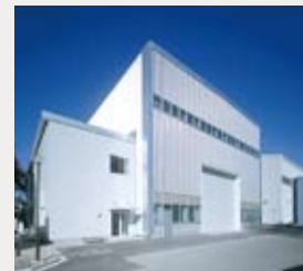
Fire protection engineering laboratory
