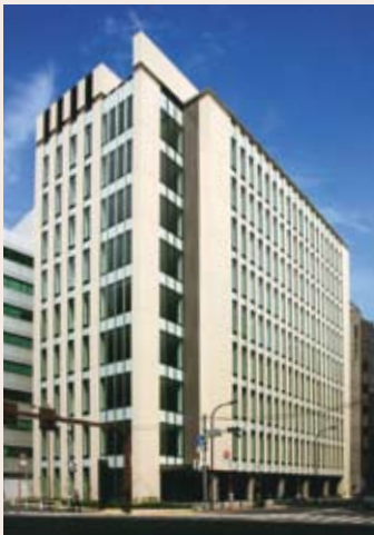
Location: Chiyoda-ku, Tokyo Site area: 1,056 m 2 Floor area: 7,931 m 2 Structure/Scale: Steel construction (partial steel reinforced concrete); 9 stories above ground
