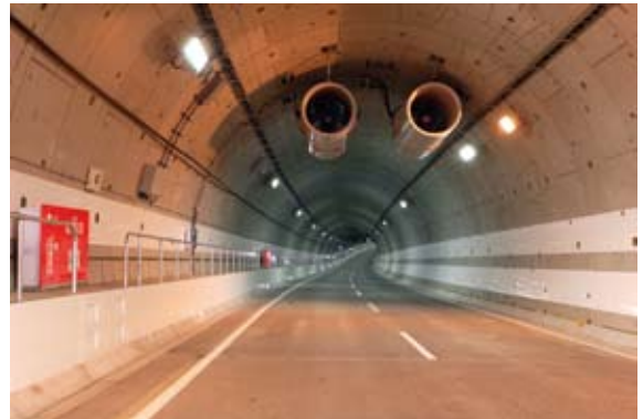
Hanshin Expressway Inariyama Tunnel ('09) Location: Kyoto
