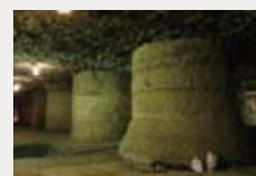
Building foundations before retrofitting
