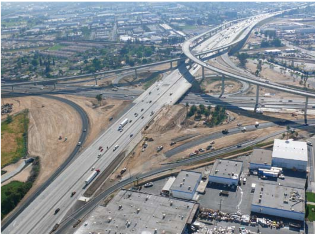
60/91/215 Corridor Improvement Project ('08) Location: Riverside, California, U.S.A.
