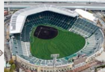
The "Silver Umbrella" roof after replacement
