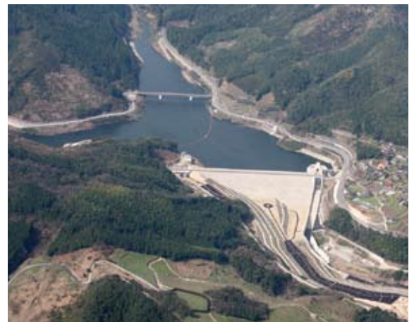
Fujinami Dam ('09) Location: Ukiha, Fukuoka
