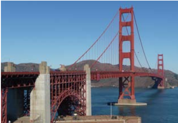
Golden Gate Bridge Seismic Retrofit ('08) Location: San Francisco, California, U.S.A.
