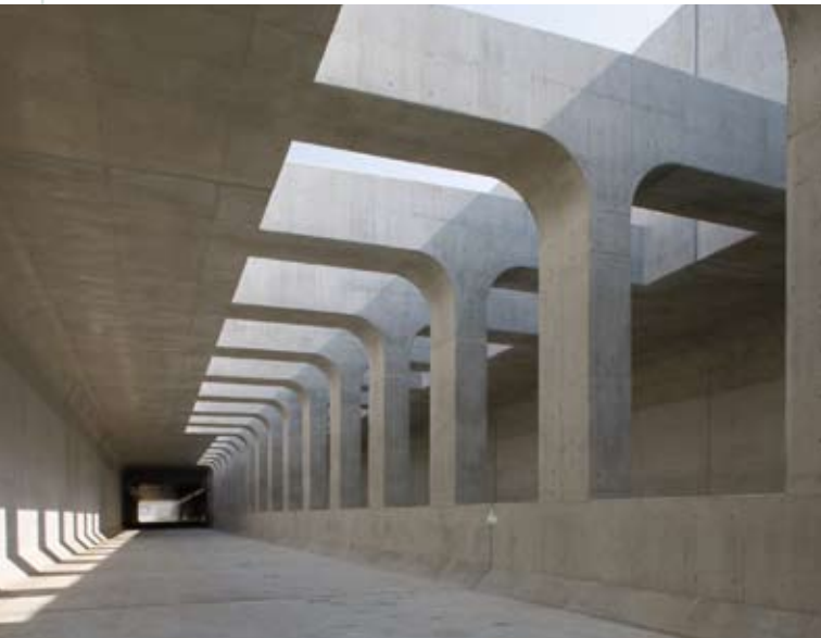
Higashi Meihan Expressway Hirabari Excavation Tunnel ('09) Location: Tempaku-ku, Nagoya
