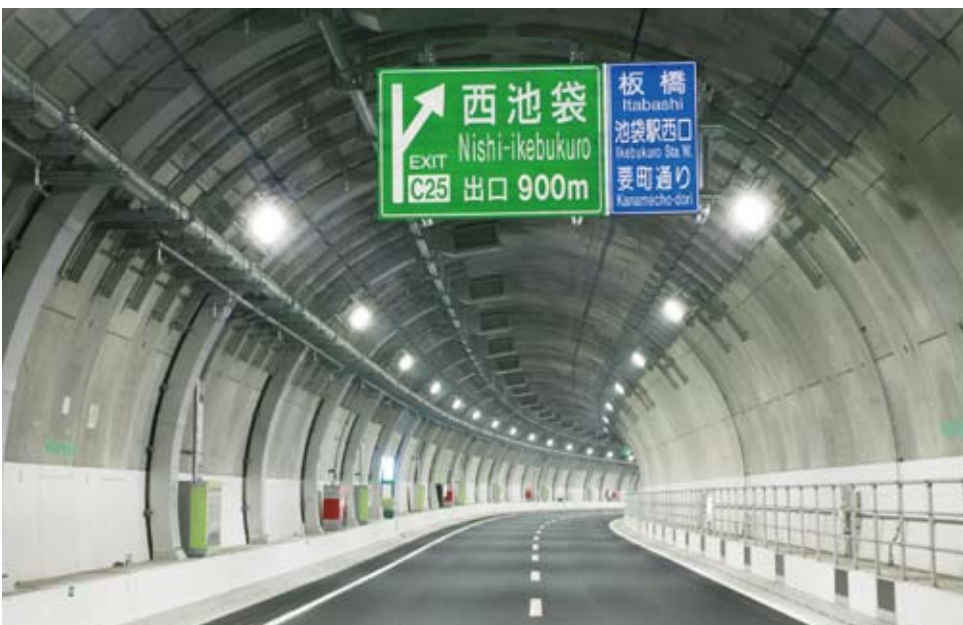
The Metropolitan Expressway Central Circular Yamate Tunnel Naka-Ochiai Shield Tunnel (outbound) ('07) Location: Toshima-ku and Shinjuku-ku, Tokyo
