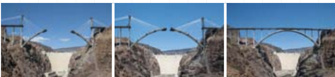
Construction of the arch (Hoover Dam is visible in the distance)
