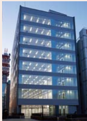
Mito North Front Building (Mito, Ibaraki)
