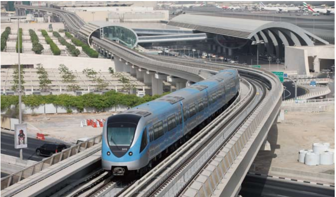
Dubai Metro Red Line ('10) Location: Dubai, United Arab Emirates
