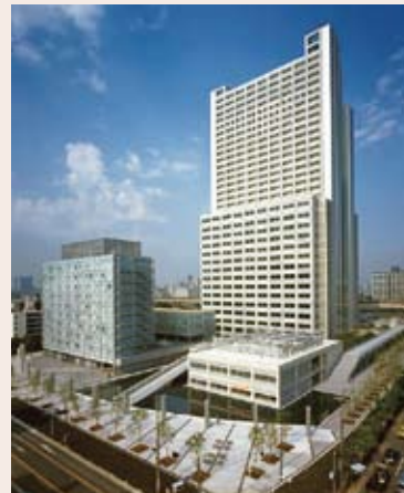
Location: Sumida-ku, Tokyo Site area: 23,124 m 2 Floor area: 103,709 m 2 Structure/Scale: Steel construction (partial reinforced concrete, steel reinforced concrete); 33 stories above ground, 2 stories below ground
