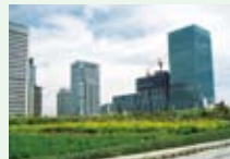
Roof greenery system
