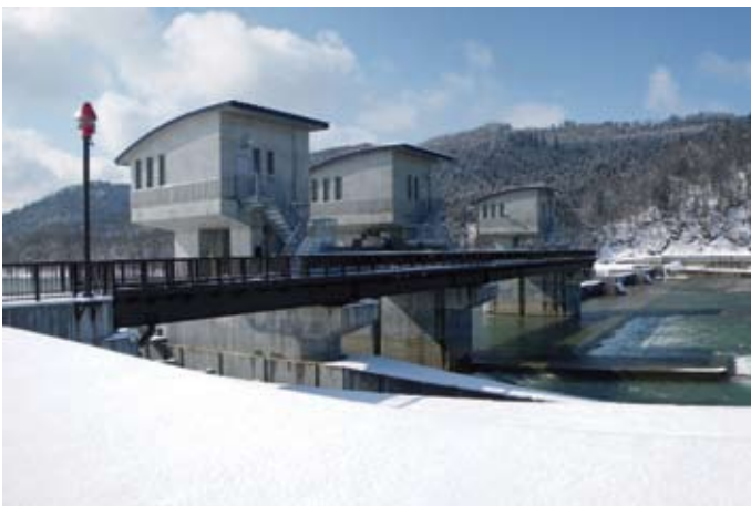
Minase Headwork* ('09) Location: Yokote, Akita
