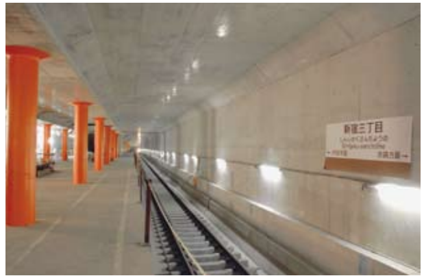
Tokyo Metro Fukutoshin Line Shinjuku 3-Chome Station ('09) Location: Shinjuku-ku, Tokyo
