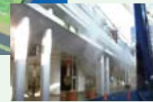
Outdoor moisture droplet cooling system
