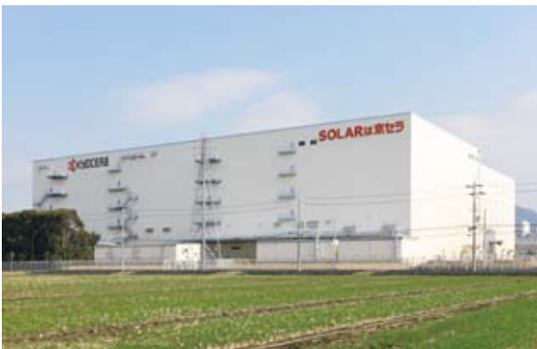
Kyocera Shiga-Yasu Factory Building No. 28 ('10) Location: Yasu, Shiga
