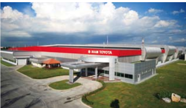
SIAM TOYOTA ENGINE PLANT NO. 2 ('09)* Location: Chonburi, Thailand
