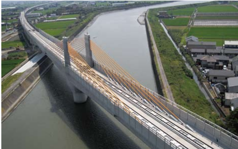
Kyushu Shinkansen Onogawa Bridge ('09) Location: Uki, Kumamoto
