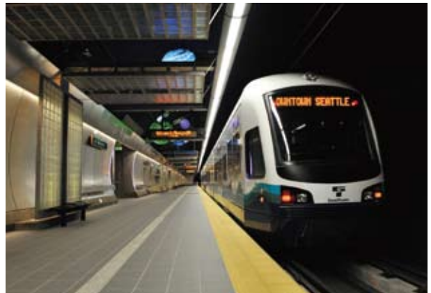
Central Link Light Rail Beacon Hill Project Beacon Hill Tunnel & Station ('09) Location: Seattle, Washington, U.S.A.
