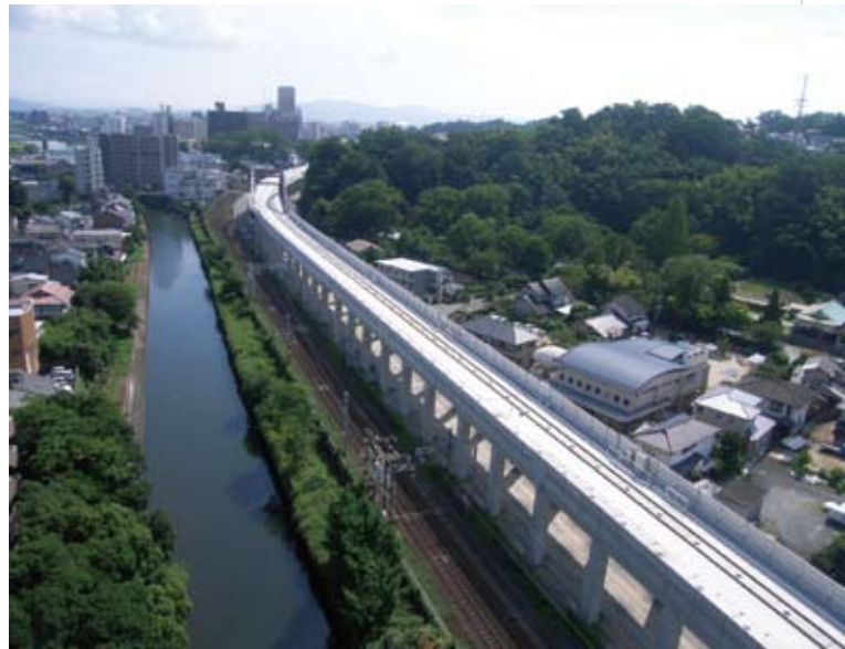
Kyushu Shinkansen Kitaoka Viaduct ('09) Location: Kumamoto, Kumamoto
