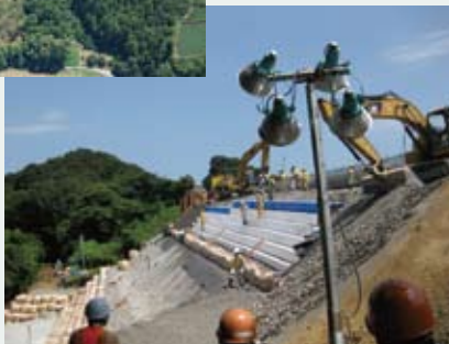
Large-bubble styrofoam reduces the surface burden
