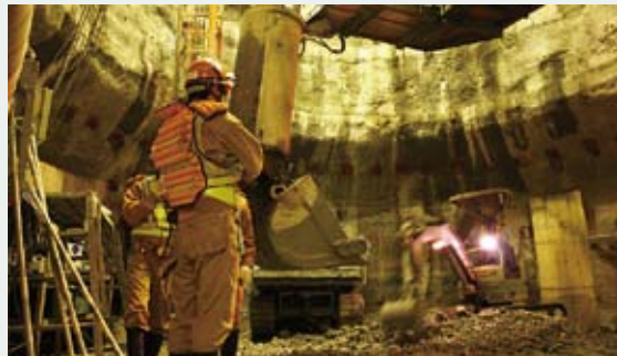
Excavation at the deepest level
