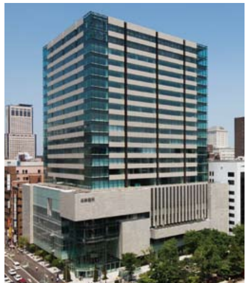
Hokuyo O-dori Center Building ('10) Location: Chuo-ku, Sapporo
