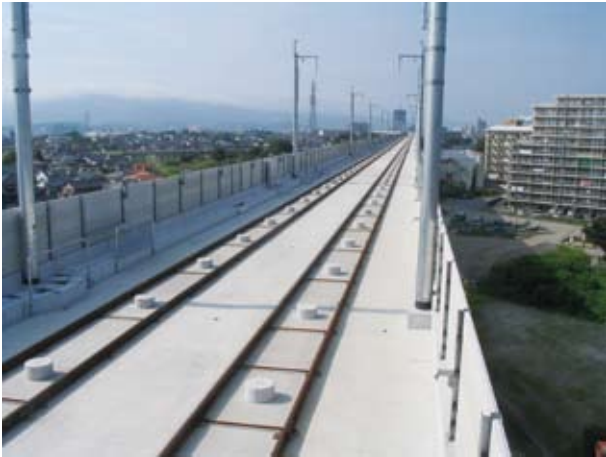
Kyushu Shinkansen Kurume-Tsubuku Nishi Viaduct ('09) Location: Kurume, Fukuoka
