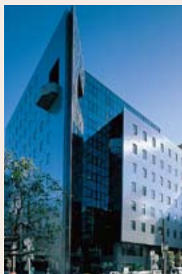
Oak Ikebukuro Building (Toshima-ku, Tokyo)
