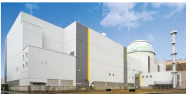
Hokkaido Electric Power Tomari Power Plant No. 3 ('08) Location: Furuu-gun, Hokkaido
