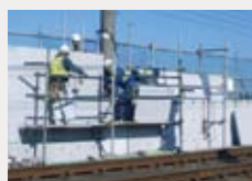
Installing a cement board
