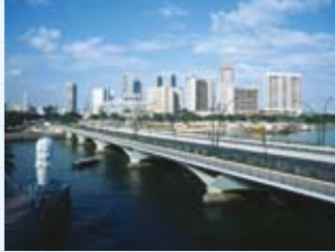
1997 Esplanade Bridge Singapore
