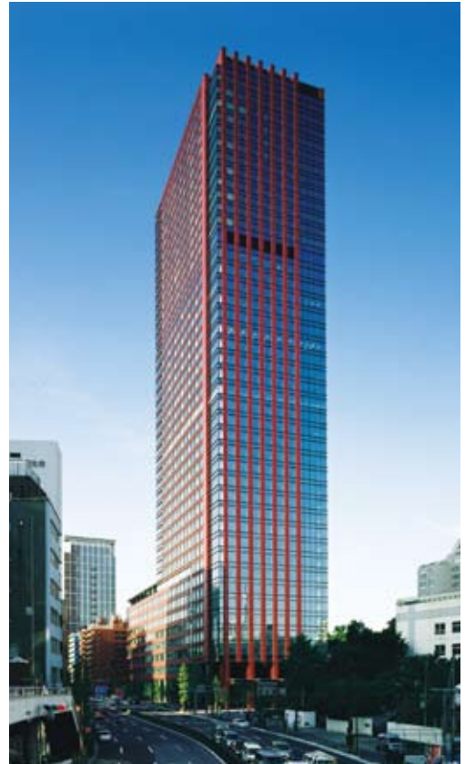
Sumitomo Fudosan Mita Twin Building West ('06) Location: Minato-ku, Tokyo
