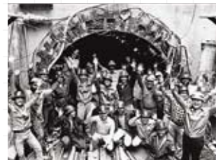
San Francisco Sewer U.S.A.
