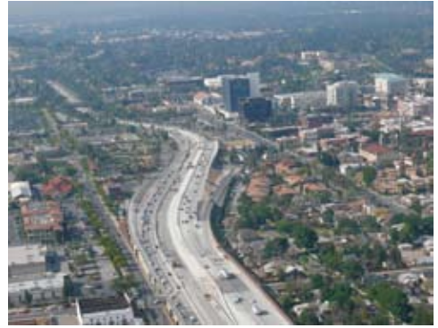
+ + 60/91/215 Corridor Improvement Project ('08) Location: Riverside, California, USA Los Angeles is the second largest city in the United States. An Obayashi joint venture was tapped to create an interchange with flyover ramps connecting Interstate Highway 215, a major traffic route on the outskirts of the city, with California state freeway routes 60 and 91, as well as for construction to expand surrounding road surfaces. Along with expanding a 16 km stretch of the project from three lanes to six lanes (a portion of which is four or five lanes), the joint venture has constructed flyovers in 15 locations. This project has reduced commuting times and lessened air pollution caused by traffic jams. + +
