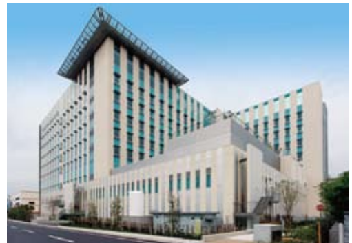
Uwajima City Hospital ('08) Location: Uwajima-City, Ehime
