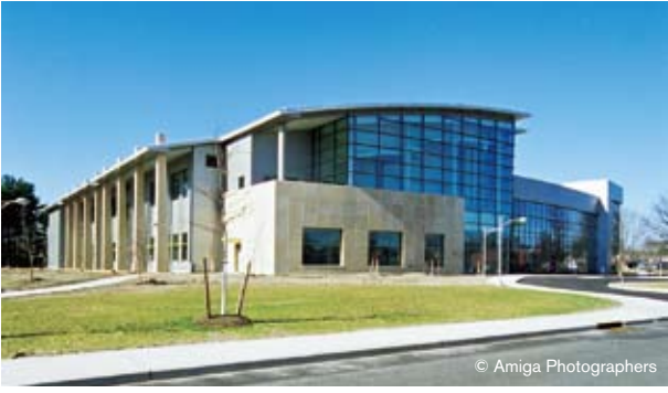
Brookhaven National Laboratory Center for Functional Nanomaterials ('07) Location: Upton, New York, U.S.A. Contractor: E.W. Howell (Obayashi Group)
