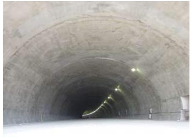
The New Tomei Expressway Kakegawa Tunnel No. 3 ('09) Location: Kakegawa-City, Shizuoka
