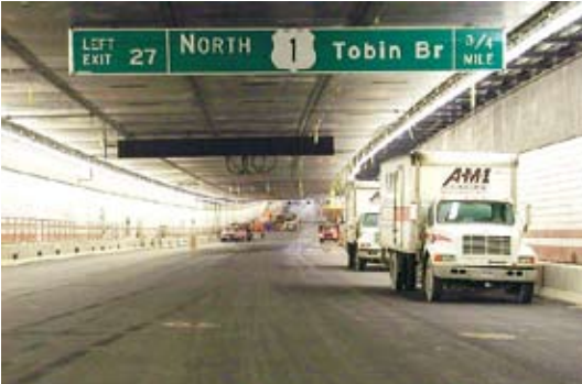
Central Artery/Tunnel Project I-93 Tunnel Finishes (C17AA) ('06) Location: Boston, Massachusetts, U.S.A.
