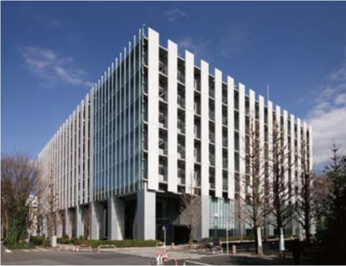
Waseda University Nishi-Waseda Campus Building 63 ('08) Location: Shinjuku-ku, Tokyo
