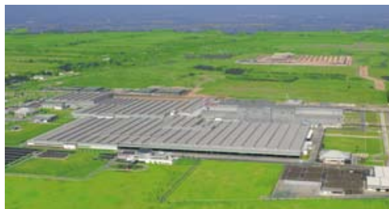
Toyota Motor Thailand Co., Ltd. Ban Pho Plant ('06) Location: Chachoengsao, Thailand Contractor: Thai Obayashi Corporation Limited (Obayashi Group)
