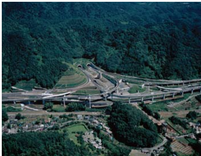
Chuo Expressway Hachioji Junction ('05) Location: Hachioji-City, Tokyo
