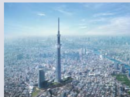
Perspective drawing of completed tower Provided by Tobu Railway Co., Ltd. & Tobu Tower Sky Tree Co., Ltd.
