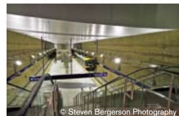
MSP LRT Tunnel and Station U.S.A
