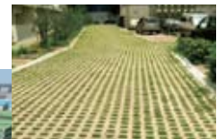
Moisture cooling system for pavement
