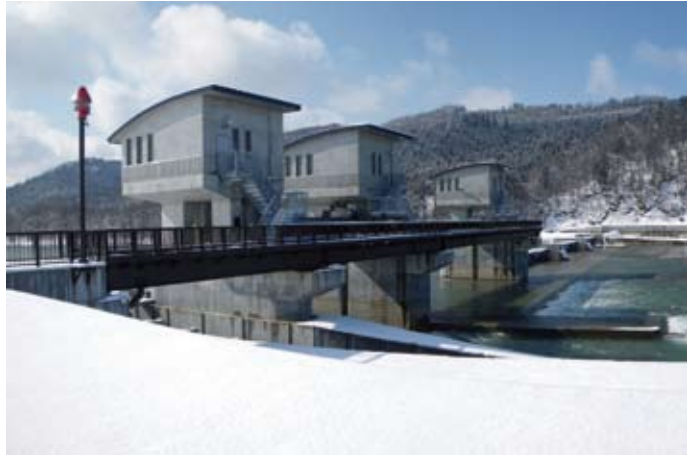
Minase Headwork* ('09) Location: Yokote-City, Akita * Headwork: A facility for taking in water from a river for agricultural use.
