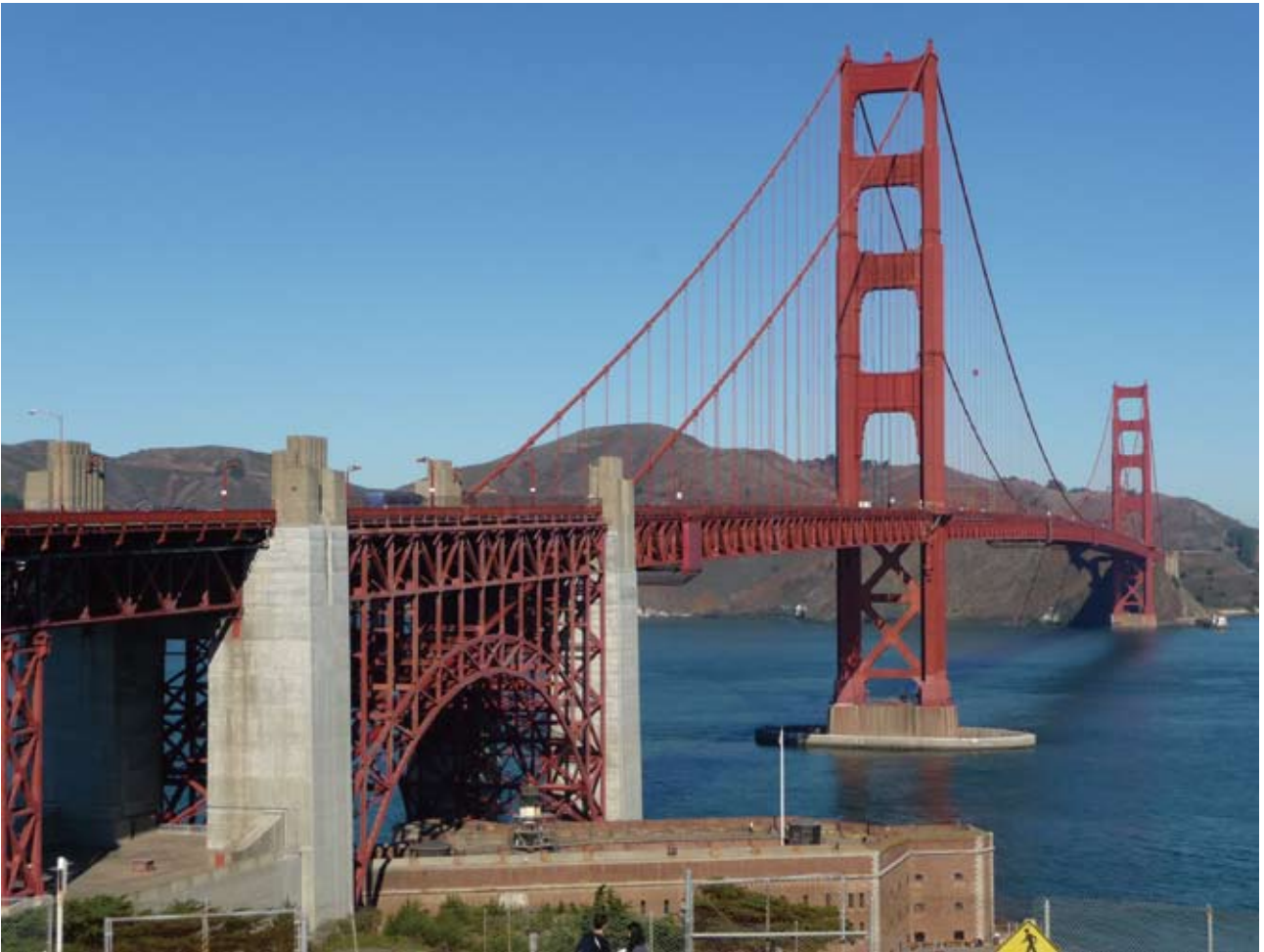
Golden Gate Bridge Seismic Retrofit ('08) Location: San Francisco, California, USA
