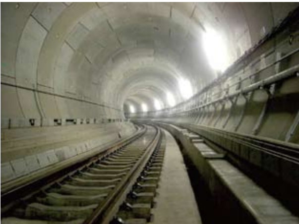
Fukutoshin Line (Tokyo Metro Subway Line No. 13) Minami-Ikebukuro Shield Tunnel (A Line) ('07) Location: Toshima-ku, Tokyo
