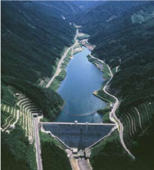
Nakakoba Dam ('07) Location: Kashima-City, Saga
