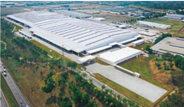
PT. Yamaha Indonesia Motor Manufacturing Karawan Factory ('08) Location: West Jawa, Republic of Indonesia Contractor: PT. Jaya Obayashi (Obayashi Group)
